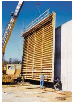
Figure 2: Temporary prefabricated form. Image from http://www.efco-usa.com/EngVer/home.html
