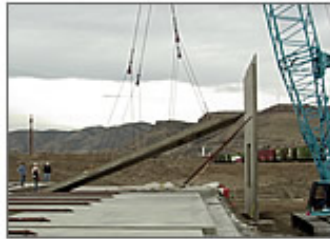
Figure 1: Pre-cast concrete wall section. Image from http://www.thermomass.com/construction/tilt.htm
